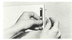
Secure the mounting strips to the rear of the cabinet panel using two screws from the hardware package.
